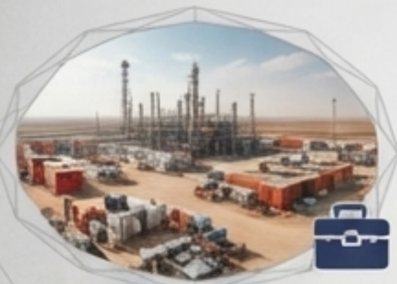
Well-mobilized Turnaround site
